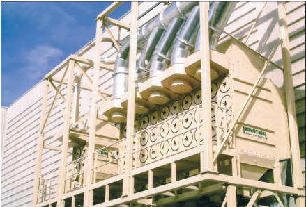
Two CDF's installed side by side at Hill AFB provide ventilation for both the recovery system and the blast room. CDF-8 on left; CDF-40 on right. Auger system transports dust to central collection area for disposal.
